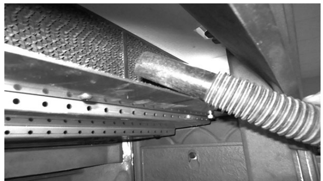
Fig. 18. Vacuum the combustor cells after brushing.
