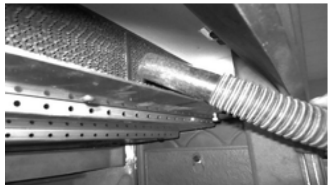
Fig. 18. Vacuum the combustor cells after brushing.
